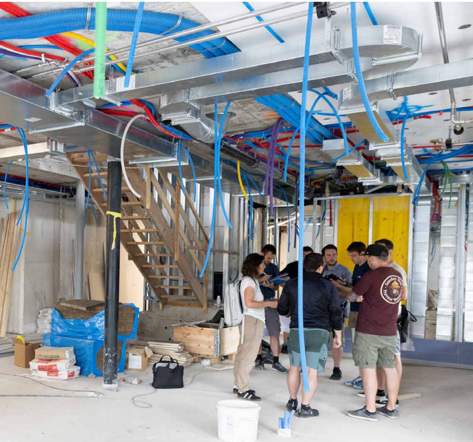
Renovation of the Guin branch
